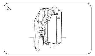
Drill the holes to a depth of 80mm using the 16mm drill bit. Afterwards, take care to ensure the concrete dust is removed from the holes.
